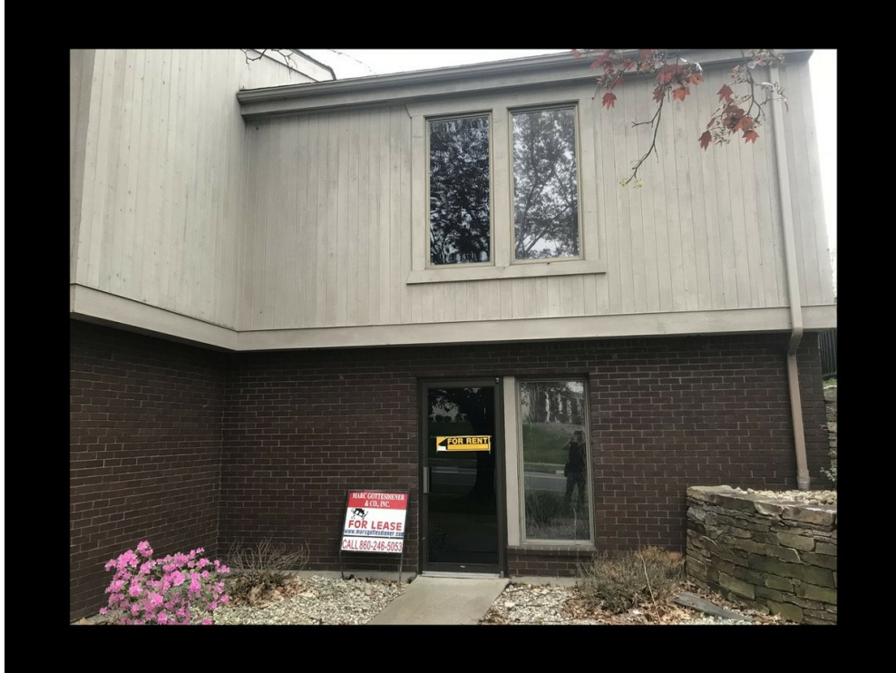
space ready-main floor
